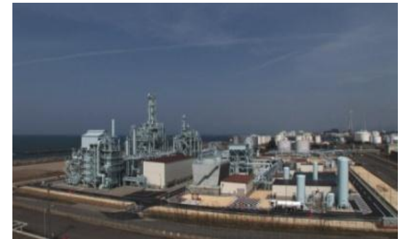
“Japan GTL” Demonstration Plant in Niigata, Japan
